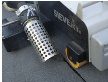
Modified bitumen welding
